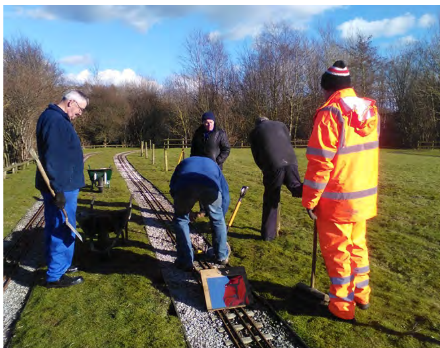
Track repair in the inside track (Sorry - none available of the outside track)
