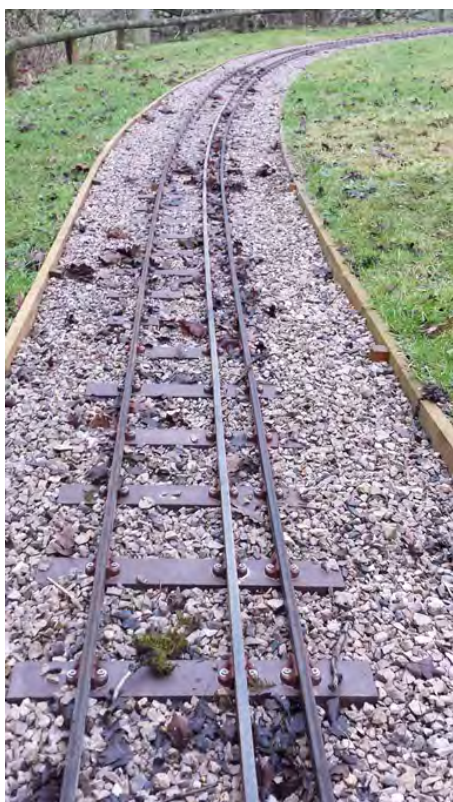
A section of the newly laid track
