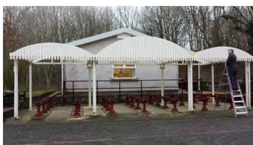
Malcolm working on the fascia
