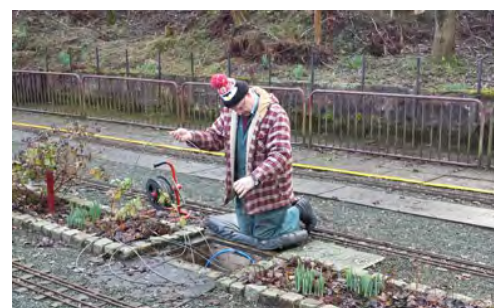
Peter installing new signalling system
